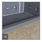
Weight is applied on and against the curb (from outside) and another 1/2" bead of sealant is applied over all curb seams and spread flat. The seams must be covered 1" either side of a seam.
