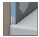
A bead of wedi Joint Sealant is applied against the tub's flange.
