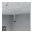
Install the ceiling suspension systems to the existing ceiling by using dowels and set the desired suspension height.
