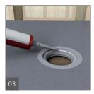
Set up a continuous 1/4" bead of wedi Joint Sealant along the top side of the wedi Fundos' valve groove profile.
