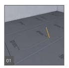
Draw ducts/grooves onto the wedi Building Panel for installation of the heating system.
