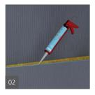
A continuous 1/2" bead of wedi Joint Sealant is applied on the foam edges of a wedi Building Panel before another panel is joined by butting tightly.
