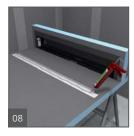
Use wedi Joint Sealant if you choose to install the optional stainless steel plate (which works with the use of Discreto's finished stainless steel drain cover).
