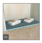
Press the Fundo firmly into the thinset bed, ensuring that the installation is level and void free. Apply some weight equally and for at least 30 minutes (thinset bags or tile boxes).
