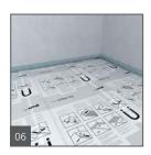
Apply a continuous 1/2" bead of wedi Joint Sealant along all seams and spread flat with a putty knife over the joints.
