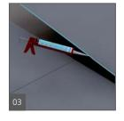
Set building panels into position using wedi joint sealant
