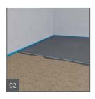
Apply the Building Panel by laying the panels into the mortar. Stagger all panel joints.
