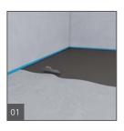
Make sure the concrete floor is even, fully cured and free of debris, oil or waxes. The wedi Building Panels are installed using modified thinset mortar using a 1/4" x 1/4" notch trowel.
