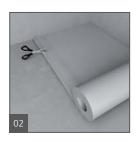
Cut Subliner Dry & Flex Pro to length. Leave the sheet a few inches longer on either end so that the membrane's adhesive layer can contract upon floor contact. Once settled in position you can cut away excess membrane.
