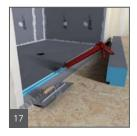
A continuous 1/2" bead of sealant is set into the channel and along the vertical curb notch part. A circle of 1/2" sealant bead is set against the wall panels where the curb attaches. A 1/2" x 1/2" bed of thinset mortar is applied to the subfloor and a skim coat on the bottom surface of the curb as a best practice. The tightly fitting curb is pressed into the connection area.
