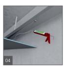
When installing wedi Building Panels to metal stud ceiling framework, use wedi Joint Sealant in addition to wedi Self Tapping Screws and Washers.
