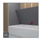
Attach a notched panel to the framework with a 1/2" bead of wedi Joint Sealant between the notch and flange. Attach the panel to the framework using wedi Washers and Screws at a rate of 1 every 12 inches along the studs. Leave a gap of 1/8" between tub edge and wedi panel bottom end to allow for movement of the tub. Alternatively apply a bead of wedi Joint Sealant in between both materials.
