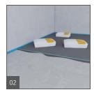
Stagger all joints when laying wedi Building Panels on the floor. Apply some weight on the boards during initial thinset setting time and especially over board transitions.
