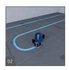
Cut grooves using a router. Cutting width should be the same as the pipe width; cutting depth should be at least 1/8" deeper. Make sure at minimum a remaining wedi panel foam thickness of 1/4" remains intact below the pipe.
