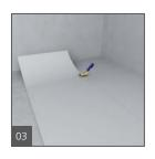
Line up sheets butted tightly but with no overlap between sheets. Seams do not require any taping or reinforcing.
