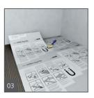
Place wedi Subliner Flex edge to edge – with the printed side facing upward – and press by using a rubber roller or wooden wedi float.
