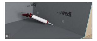
Apply continuous 1/2" beads of sealant between all connections of panels and install with tightly butted seams. Excess sealant must be spread flat with a putty knife. All seams and fastener heads in the assembly are covered with a secondary 1/2" bead of sealant and spread flat. The seams should be covered 3/4" to 1" on either side of seam. All fastener/washers are covered with sealant stretching 1" over the washer edges.
