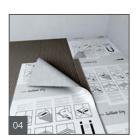
The sheets must overlap 2" at joints/transitions. Apply a bed of thinset mortar with the flat side of the trowel onto the lower mat joint connection area and press flat.
