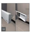
The unit is now installed and a double wall or seat/shelf unit can be installed around it, integrating the unit. The installation instructions show in detail how to insert and adjust the drain cover which can be reversed from finished surface to tileable surface. Adjustments can accommodate thickness of floor and wall tiles before fixing its position.
