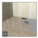
Apply a skim coat and finally a combed through bed of a thinset using modified thinset ANSI 118.4 and 1/4" x 1/4" notch trowel.
