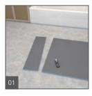
Measure and cut wedi Building Panel to fit the 16 inch o.c. framework (wood or metal). Notch out all panels if installed around the perimeter of a flange tub to integrate the flange and achieve a plumb wall with square and tight corners.
