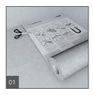
Lay out wedi Subliner Dry and cut to size using a knife or scis-
