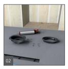
Assemble the drain unit following the instruction drawing. wedi's Riolito bases can be cut to size on all sides making drain positions close to the wall possible. Please do not cut into the linear drains plastic flange integrated into the coated foam part of the base. Once cut the 1/2" x 1/2" channels at the new base perimeter must be re-established. When cutting close to the drain channel always leave enough wedi foam for re-making the needed 1/2" x 1/2" channel.
