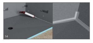
Apply continuous 1/2" beads of sealant between all connections of panels and install with thigthly butted seams. Excess sealant must be spread flat with a putty knife. All seams and fastener heads in the assembly are covered with a secondary 1/2" bead of sealant and spread flat. The seams should be covered 1" on either side of seam. All fastener/washers are covered with sealant stretching 1" over the washer edges.
