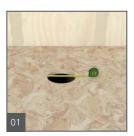
Cut the 2" pipe flush (or max. 1/8" above) to the floor construction. Make sure that the cut out fits to the Fundo panel drain. Cut out a 5" diameter hole around the 2" pipe to allow the wedi drain to be inserted into the subfloor while the cut out area must remain free of deflection. The drain and trap have to be sturdily fastened to the sub floor.
