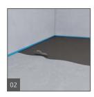
The panels are installed in a full coverage setting bed using modified thinset mortar allowing best connection between subfloor and wedi panel.
