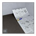
Insert wedi Subliner Dry with the printed side facing upward and press on with a rubber roller or wooden float.
