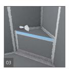
thinset mortar and alkali resistant fiberglass mesh tape by wedi, applied over this seam. Alternatively, benches and seats are offered as prefabricated units made by wedi. For longer or larger benches built from our 2" building panel, always install one spacer every 18" in either direction.
