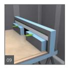
Apply some temporary weight against the metal plate so the sealant can set.
