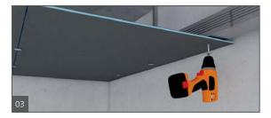
Screw wedi Building Panels to framework using either wedi Wood Screws and Washers (wooden frame) or wedi Self Tapping Screws and Washers (steel framework). The fastener pattern is 1 fastener per every 6 inches. Make sure to always use washers/fasteners in panel seams to ensure smooth transitions.
