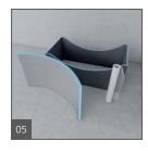
Once the thinset mortar has set, the shaped wedi Buiding Panel can be moved into its intended final position or application.
