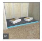
Press the Fundo firmly into the thinset bed, ensuring that the installation is level and void free. Ensure wedi drain's sealing gasket is firmly inserted in the wedi trap with no chance that thinset could have pushed into this connection area. Apply some weight equally and for at least 30 minutes (thinset bags).
