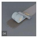
Tape all joints with wedi fiberglass mesh tape in dry areas or wedi Waterproof Sealing Tape or wedi Joint Sealant in wet areas. Fastener locations should be waterproofed too using wedi Joint Sealant. Begin tiling!
