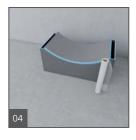
... and apply wedi Self Adhesive Mesh Tape followed by a flat application of thinset mortar
