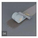
Tape all joints with wedi fiberglass mesh tape in dry areas or wedi waterproof sealing tape or wedi Joint Sealant in wet areas. Begin tiling!
