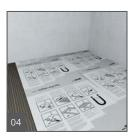
Remove any escaping mortar and/or air bubbles. Do not overlap.
