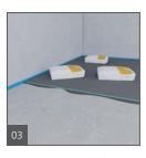
Stagger all joints when laying wedi Building Panels on the floor. Apply some weights such as tile boxes equally distributed over the wedi panel surface.
