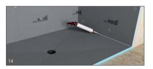
Apply continuous 1/2" beads of sealant between all connections of panels and install with thigthly butted seams. Excess sealant must be spread flat with a putty knife. All seams and fastener heads in the assembly are covered with a secondary 1/2" bead of sealant and spread flat. The seams should be covered 1" on either side of seam. All fastener/washers are covered with sealant stretching 1" over the washer edges.
