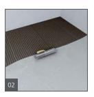
Apply modified thinset mortar onto a suitable, even, loadbearing and clean subfloor using a 1/4" x 1/4" notch trowel.
