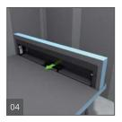
Place the Fundo Discreto unit over the channel/drain unit. Joint sealant will adhere the unit to the base.
