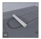
Apply wedi's wide self adhesive reinforcement tape over the installed ducts. Start tilling. Tiles smaller than 4" x 4" should not be used over hydronic system installation surfaces.
