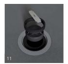
Tighten (squeeze) the rubber caulking gasket firmly with the caulking nut (use a flat headed screwdriver) and finally insert the plastic frame and strainer on top (without adhesive). The frame and drain cover will be held in a grout joint only once tiling commences.
