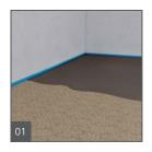
Simply spread modified thinset mortar over a clean wood subfloor using a 1/4" x 1/4" notch trowel provided the subfloor is even and loadbearing.
