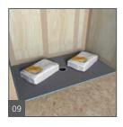
Press the wedi Fundo Ligno firmly into the thinset bed, ensuring that the installation is level and void free. Apply some weight equally and for at least 30 minutes (thinset bags).
