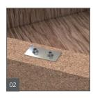
Where fixtures are integrated into the tub deck structure, they should be equipped with a stainless steel plate fixing their position
