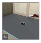
Set up a continuous 1/2" bead of wedi Joint Sealant along the pans channel on the outer perimeter and only in areas where you can immediately install a building panel into the fresh sealant.
