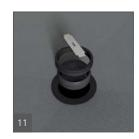
Tighten (squeeze) the rubber caulking gasket firmly with the caulking nut (use a flat headed screwdriver) and finally insert the plastic frame and strainer on top (without adhesive). The frame and strainer will be held in a grout joint only once tiling commences.
