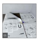
Press on the overlapping area with a trowel or rubber roller. Remove any escaping mortar and air pockets. Cross joints should be avoided.
