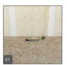
Cut the 2" pipe 1 1/4" below the top of the Subfloor. Use the oval shape cutting template to cut subfloor using a jigsaw to allow wedi drain trap to be inserted and connected to floor pipe using appropriate ABS compatible or multipurpose cement glue. Please also check cement glue compatibility to floor pipe material. The drain and trap have to be secured to the subfloor. Drain recess cut out must not add deflection to subfloor.
