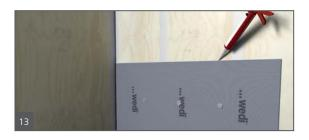
Push the wedi panel all the way into the channel of the shower base channel and its bead of sealant. Smooth out any pushed out sealant on inside seam using a putty knife. Fasten the panels directly to the studs starting 1 ft above the base and at a rate of 1 fastener per 1ft. One extra fastener is set into the seam to the next panel to create a flush transition.
