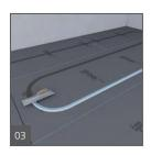
Install tubing into the groove. Fill tile adhesive into the pipe duct to cover pipe and fill voids.
