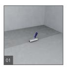
Prime all suitable, even,loadbearing and clean subfloors and wait until wedi Primer Pro is tacky to the touch. Make sure there are no contaminants or older seals on subfloor (Primer Pro will get flaky/no adhesion). Make sure subfloor is not too porous (if concrete) so it will absorb all primer but will not allow for a consistent primer film as needed.
